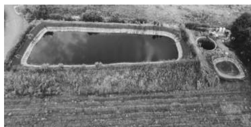
AERIAL VIEW OF RAIN WATER RESERVOIR AT SULA
